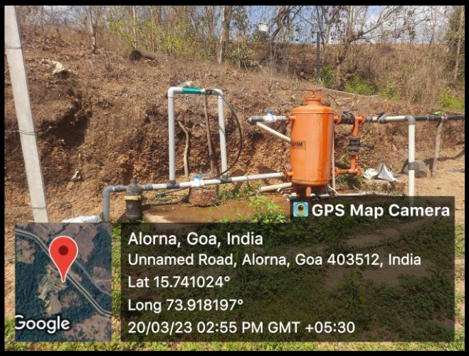
Drip Water Filtration Unit
