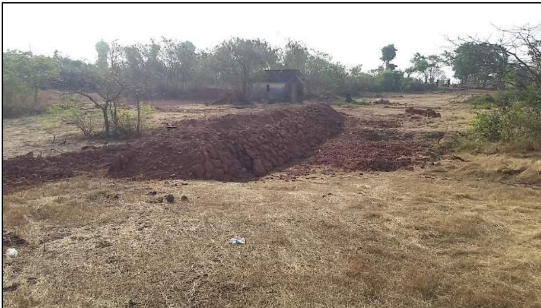
Figure 6.9 : Water harvesting bandhara(bandh) implemented. (Front view)
