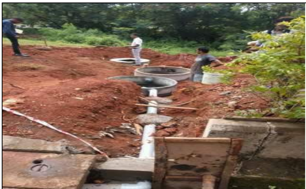
Figure 6.5 : Installations of Siltation, Filtration Chamber and Borewell Pits
