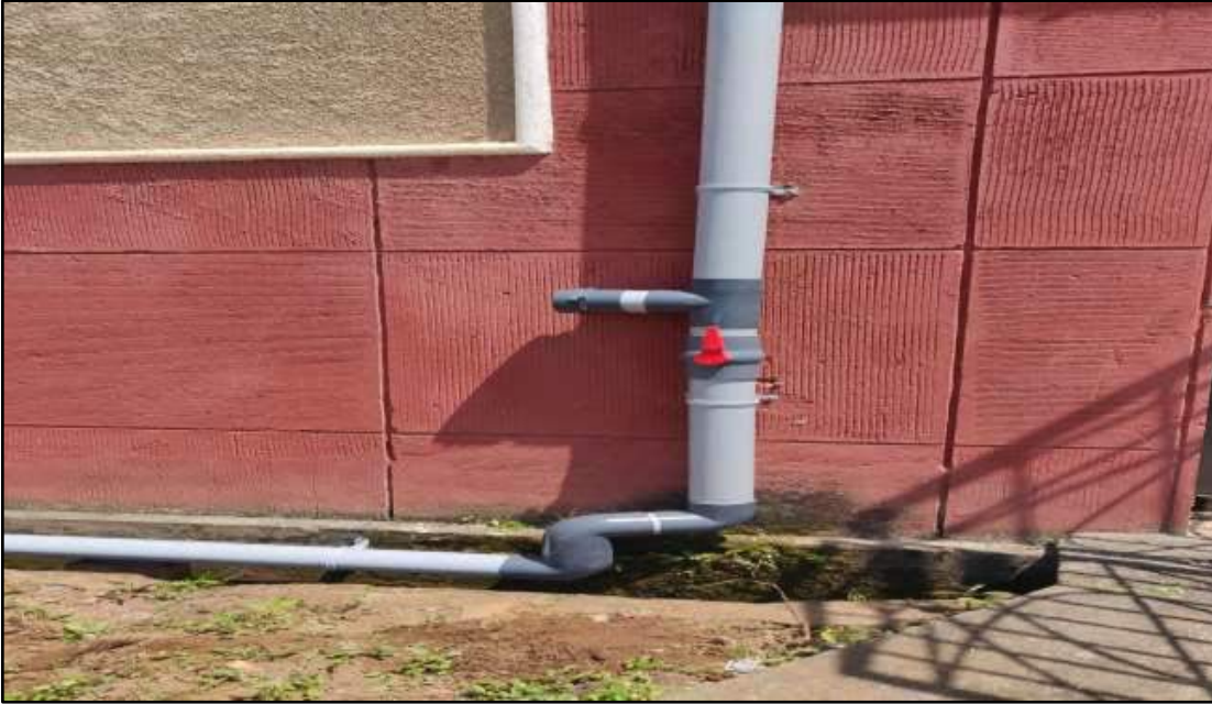
Figure 6.7: School of Chemical Science building under rainwater harvesting piping Connections from Roof for downtakes
