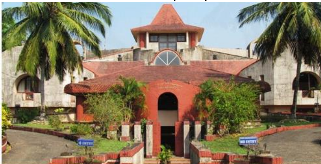
Goa University Administrative Office
